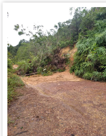
Landslide blocking roads at Hamalidah's village
